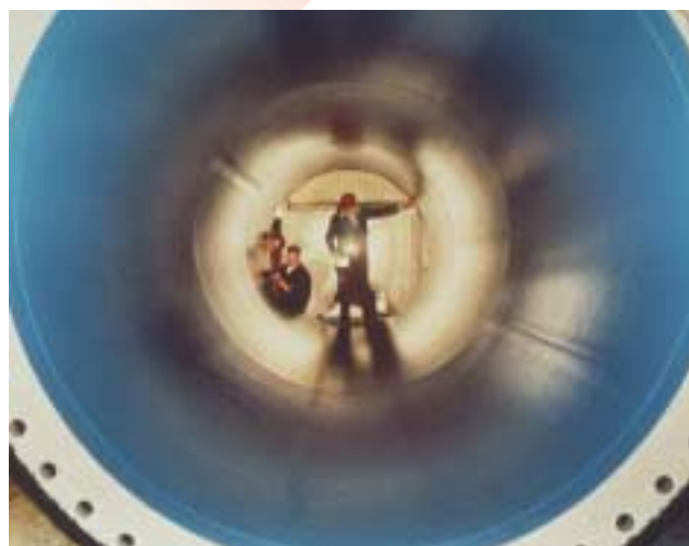
Internal lining to improve flow rates.
