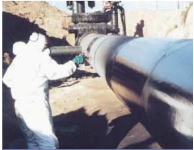
Solution - Rehabilitation with Acothane.
